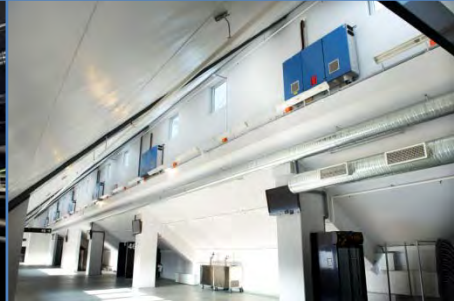
Swedbank Stadion, Malmö
